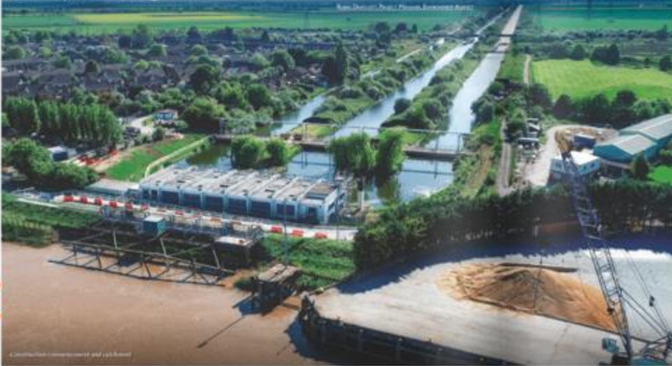
Construction commencement and early work
